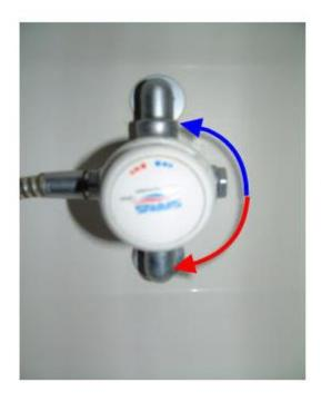
To increase the temperature turn the main body of the shower unit, the further you turn the control the hotter the water temperature. As a guide the control indicates settings from 1-9 if you feel the temperature is too hot or only warm at level 9 then please contact reception and ask to have the temperature checked and adjusted if necessary.
